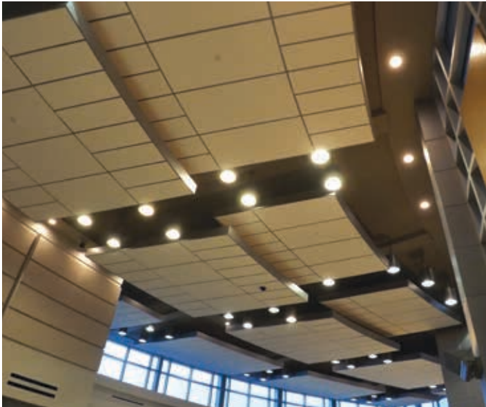
Additional after photos
